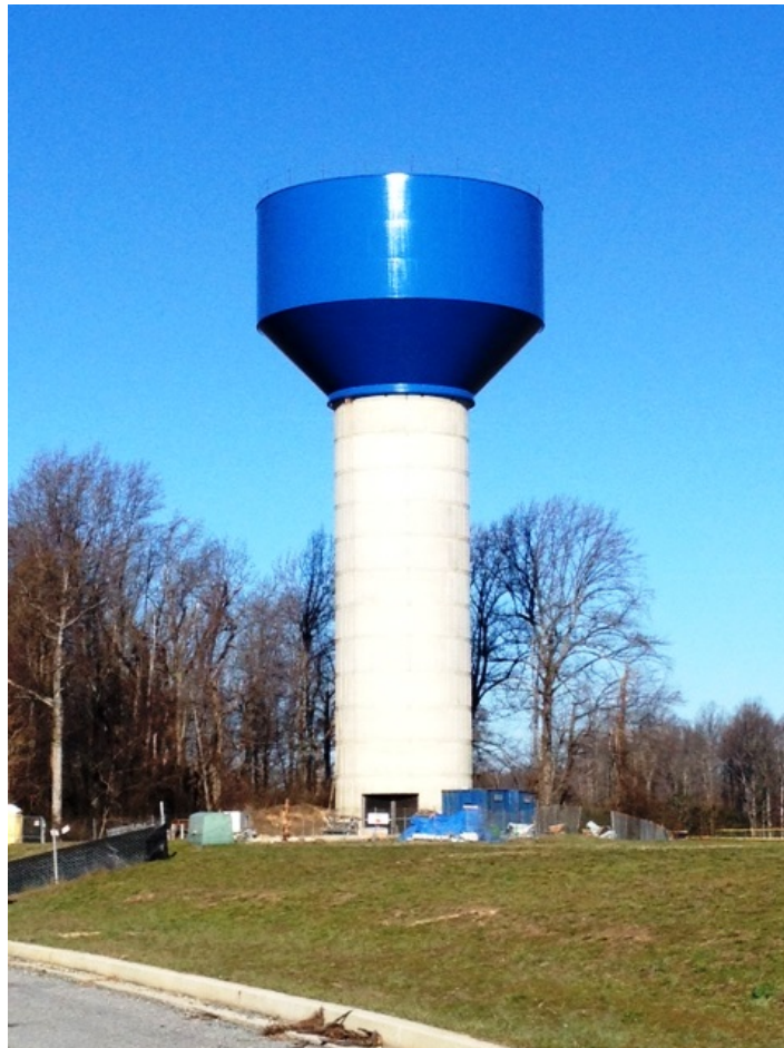
East Prince Frederick Elevated Storage Tank
